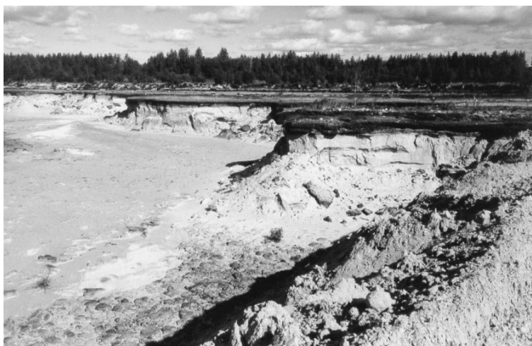
Fig. 3. Technogenic valley formed after sand flow into the trench in March 1999
